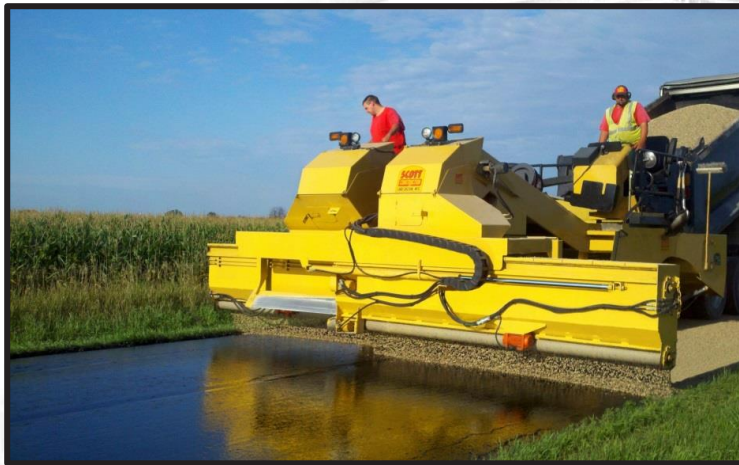
Aggregate Seal Coating
