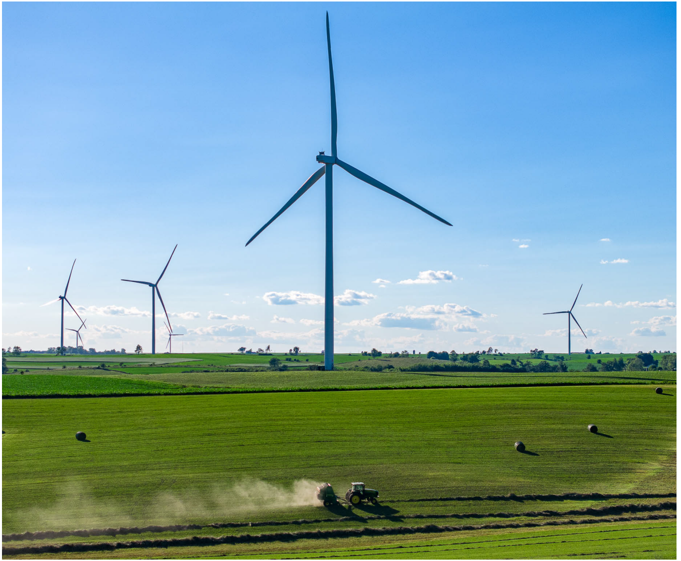
Invenergy-operated Red Barn Wind Park, located in Grant County.
