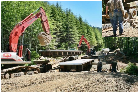
Modules set side-by-side
