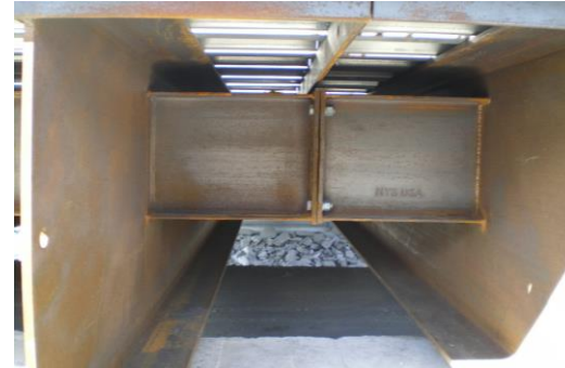
Center Diaphragms bolted together
