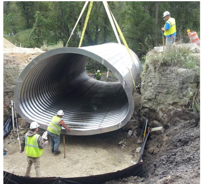
The Town of Onalaska in La Crosse County was seeking the replacement of four area bridges, however while working with GEC engineers, the Town opted to replace the bridges with culverts, at a fraction of the cost.
