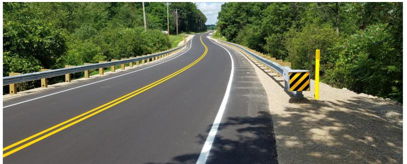
CTH H in Waushara County, Wisconsin. This WisDOT STP-Rural pavement replacement project involved approximately 4.0 miles of pulverizing and overlaying the existing asphalt pavement. Steep embankments were also addressed through grading and the addition of beam guard while minimizing impacts to adjacent sensitive resources.
