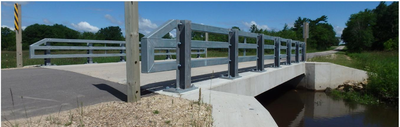
Dolphin Road over Mill Creek Bridge in Monroe County, Wisconsin. MSA was hired to design a replacement structure through the Local Bridge Program. The new structure is a single-span flat concrete slab bridge with a slight skew to better align with Mill Creek. Right-of-way impacts were avoided, which saved money for the Township.
