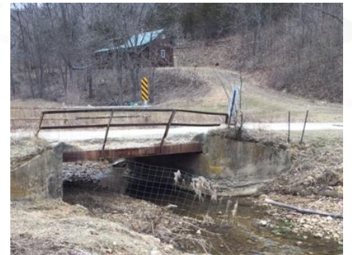
Severed East Abutment
